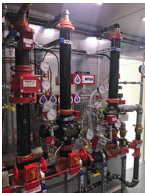
Complete standpipe system with Class I, II & III standpipes with an assortment of pressure regulating devices and hose connections ▶
