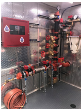
Complete standpipe system with Class I, II & III standpipes with an assortment of pressure regulating devices and hose connections ▶
