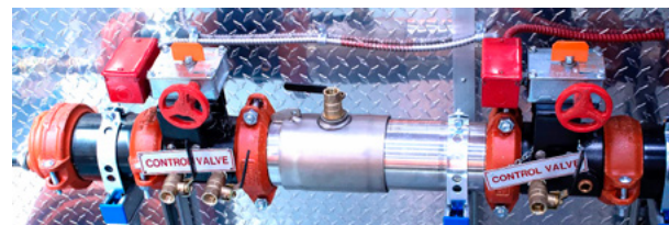
Double check valve assembly ▼
