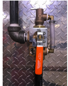
◀ Automatic air venting device
