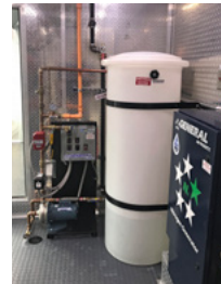
Residential pump with water tank system (NFPA 13D) ▶
