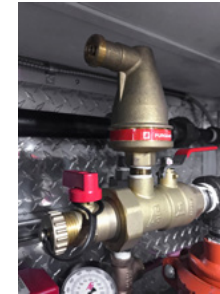
◀ Automatic air venting device
